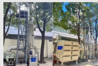
Before Replacement After Replacemen
